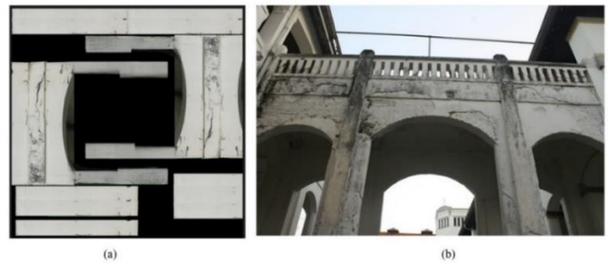
Fig. 10. Illustration of an unwrap image resulted from the 3Ds Max application program which was then applied to the warp technique in the Adobe Photoshop application program (a) using photo details of the real object (b).
