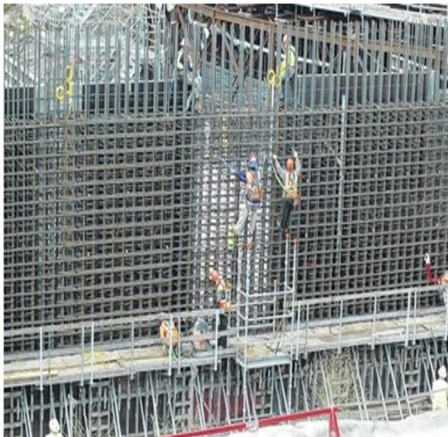
Fig. 4. Proposed workspace for the concrete wall-climbing robot
