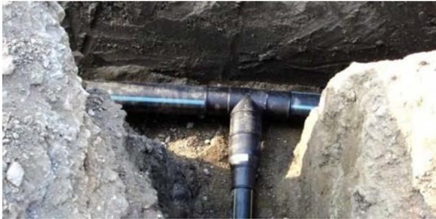
Fig. 3. Example of How a Private Branch is Actually Connected to the Distribution Pipe.
