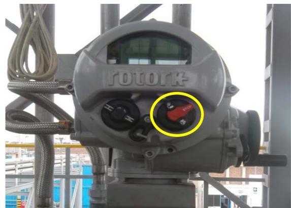
Fig. 7. Automatic Remote Actuation Switch and Scale Platform.
