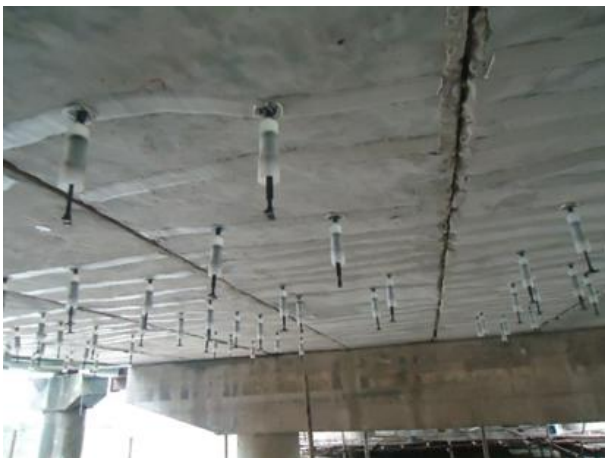
Fig. 1. Schematic diagram of concrete bridge cracks
