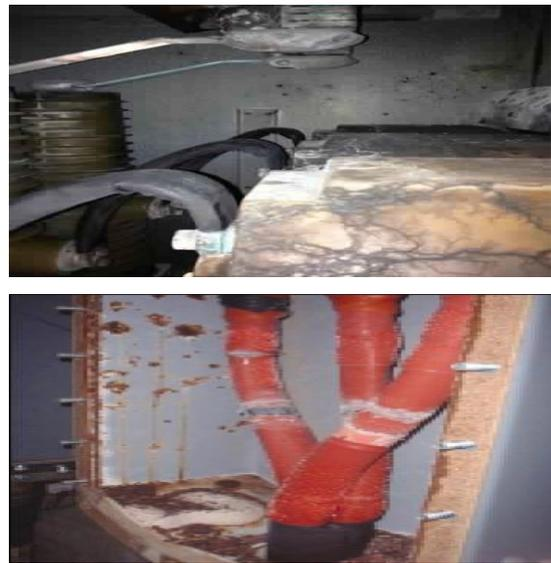
Fig. 2. Apparition of the dew inside the electric cells
