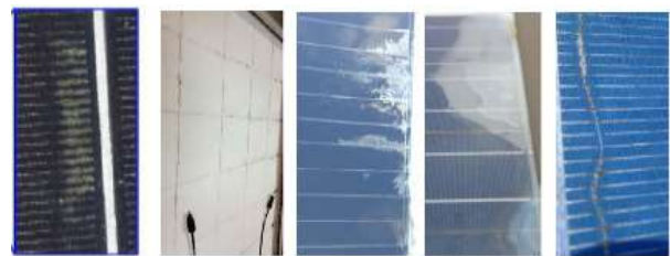
Fig. 4. Example Images [13]. A Few of the known Degradation Modes Found in PV Modules in the Field. These Modes and others are Targeted for Reproduction by C-AST Protocols. From Left to Right: Corrosion, Polyamide Backsheet Cracking, Edge Seal Failure, Delamination, Snail Trails.
