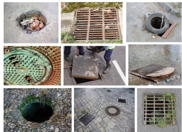
Fig. 1. Samples of varied manhole situations.
