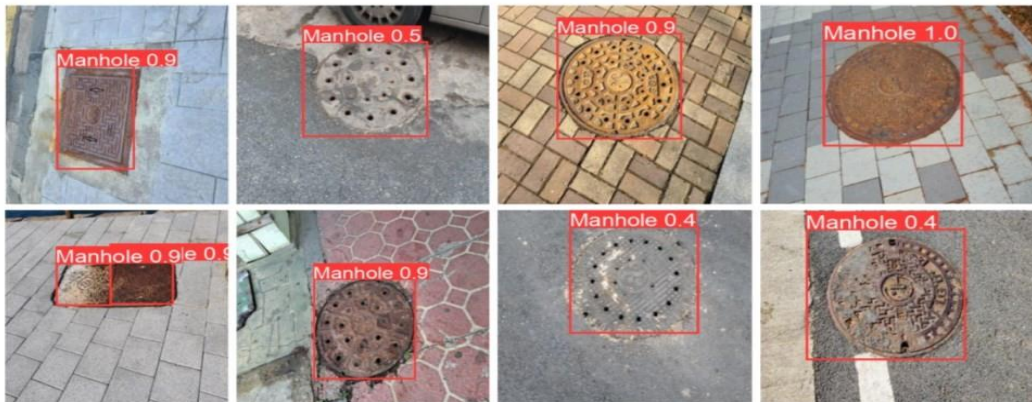
Fig. 6. Examples of good detection of manholes cover using Yolov8.
