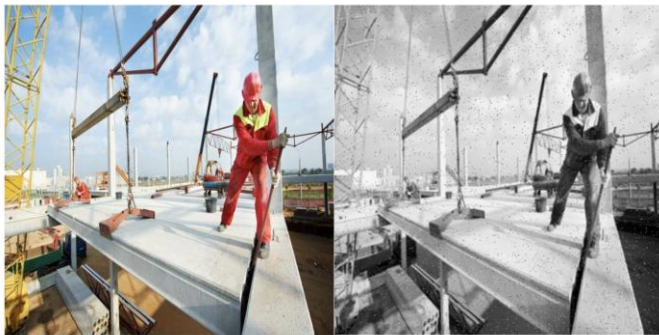
Fig. 3. Example of data augmentation added to construction site image. Original image (Left) and augmented image (Right) with 25% Grayscale, blur 4.8px, and noise 1.8px.
