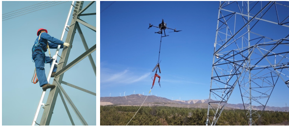
Fig. 1. The quadcopter drone operates near the power transmission tower while carrying our specially designed mounting device for fall protection lanyards.
