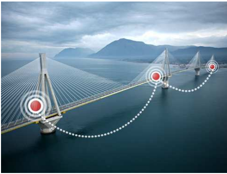
Fig. 1: wireless sensors placed on bridge [13]
